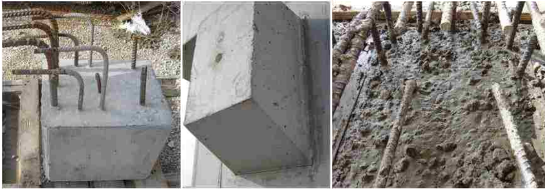
Figure 1.2. Precast button corbel - Facility #1 (left), precast button corbel in place (center), and precast button corbel - Facility #2 (right)
