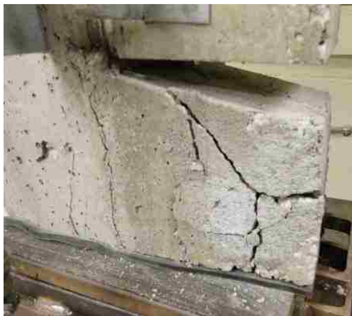
Figure 3.12. Premature flange failure
